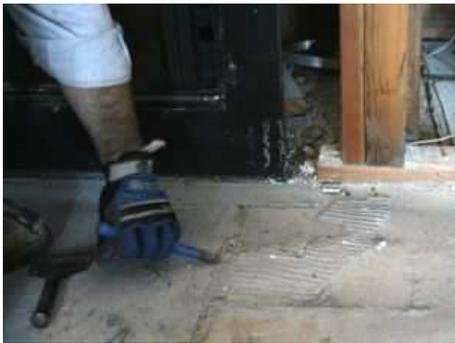
If your fireplace is a "zero-clearance" factory insert, you may find that the tile is actually just glued to gypsum drywall as in the picture above. Taking the tile off that is going to destroy the drywall, so can make your job easier by removing both simultaneously. Saw along the wall panel at the edge of the tile, and then pry the gypsum drywall/tile off together.
